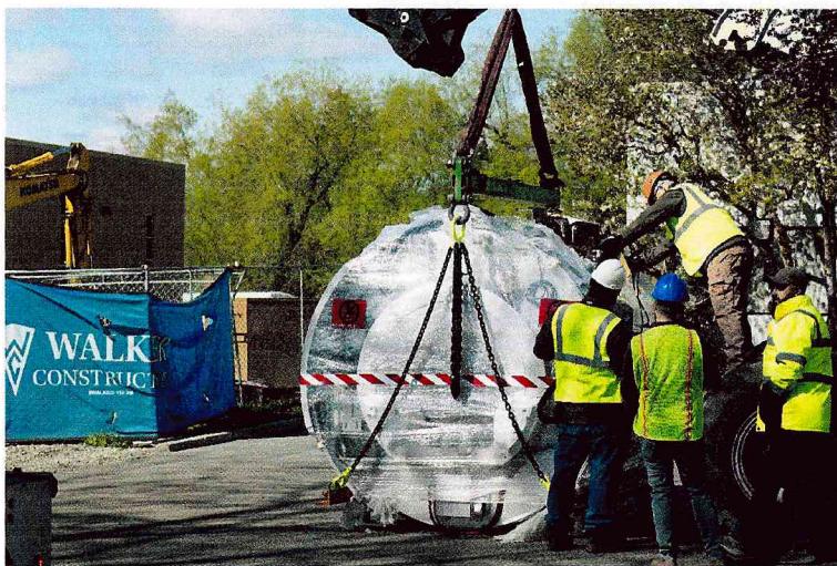
Figure 4: MRI is unloaded at KVH 4.16.24
